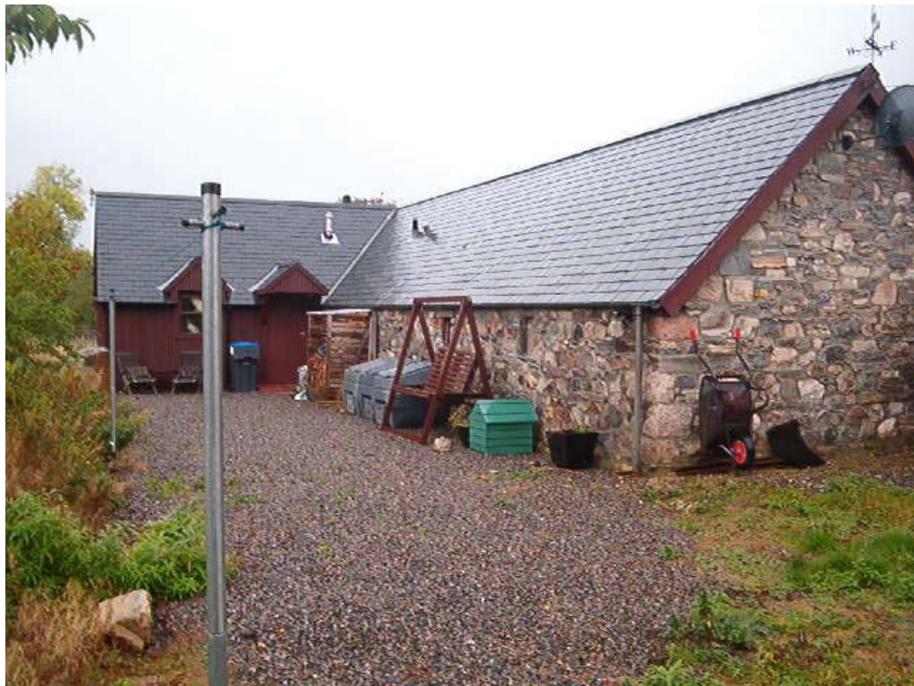
Fig. 2. Rear of Existing House with Existing Extension
