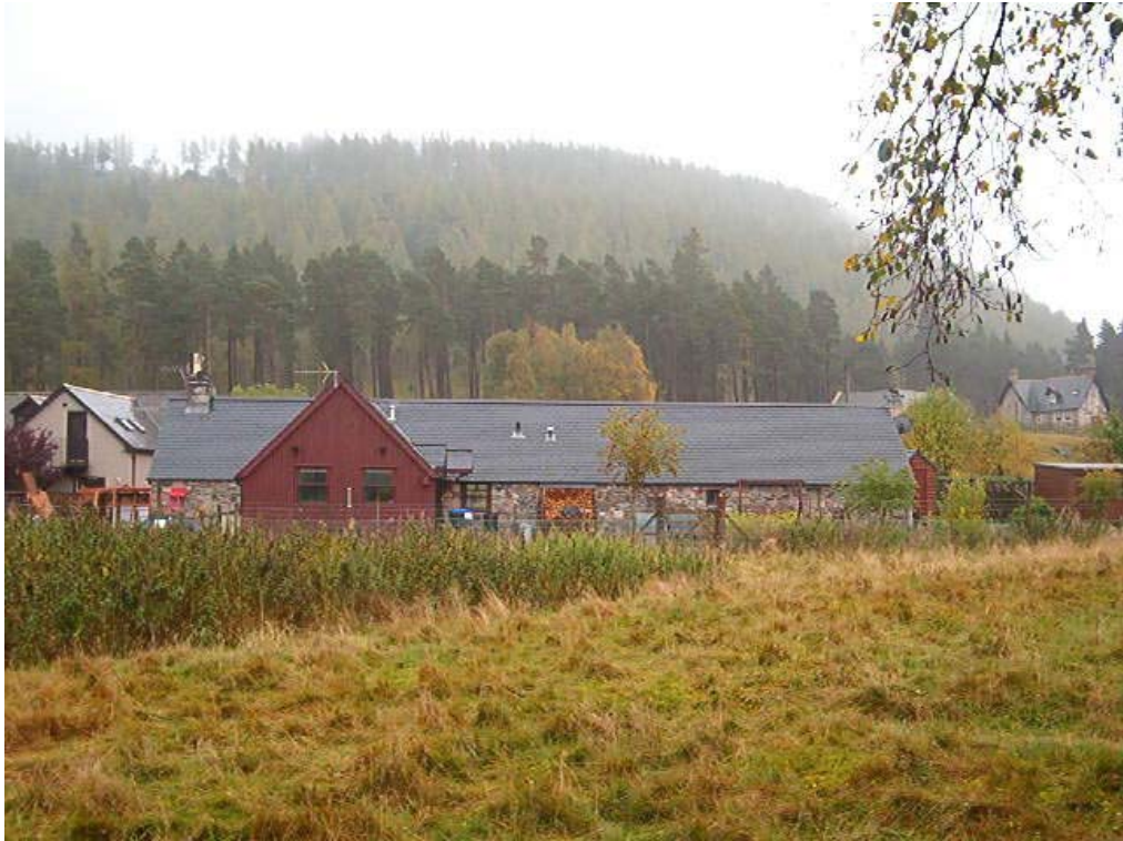
Fig. 3. Rear of Existing House Viewed from the North
